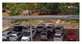
In India, two photovoltaic systems have been installed. The larger system, set up in 2019, has a capacity of 45.3 kW. The second one, which was installed in 2020, has a capacity of 25 kW. Together, these photovoltaic systems have generated 260,000 kWh of electricity since they began operating.
